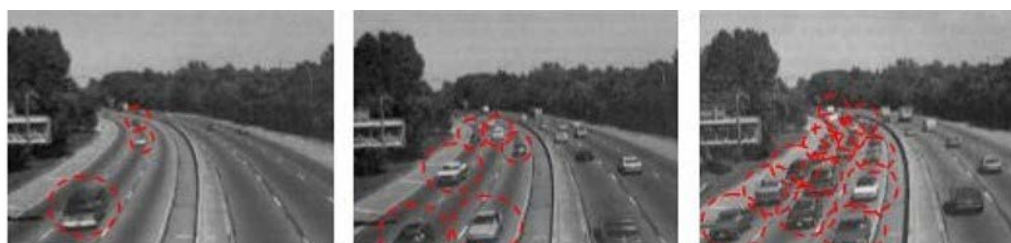
(a) Service level A (b) Service level C (c) Service level F
