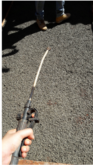
Photograph 7. Hydration of concrete.
