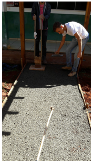
Photograph 8. Concrete hydration and compaction.
