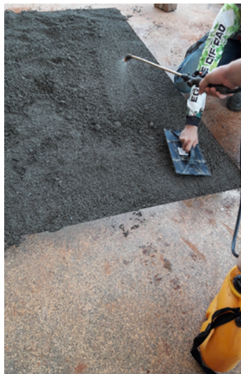
Photograph 12. Hydration of concrete hydrate it with a sprayer.
