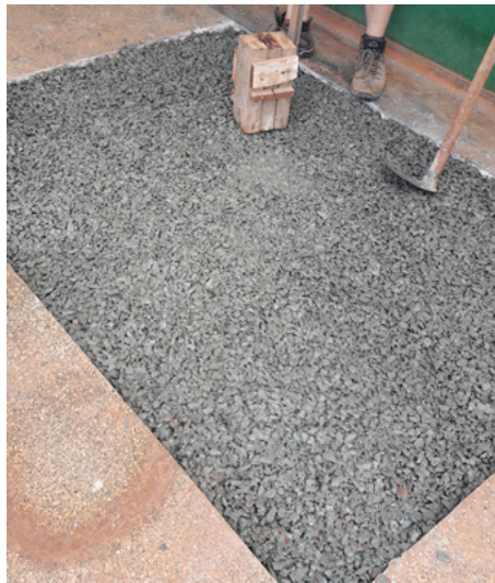
Photograph 11. Use of “soquete” to compact the concrete.
