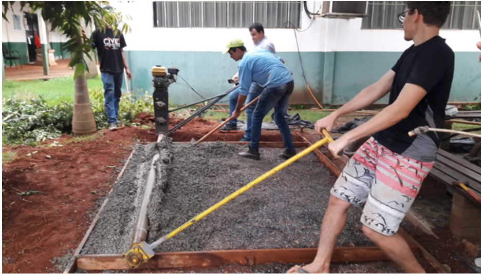
Photograph 17. The compressor roller in use.
