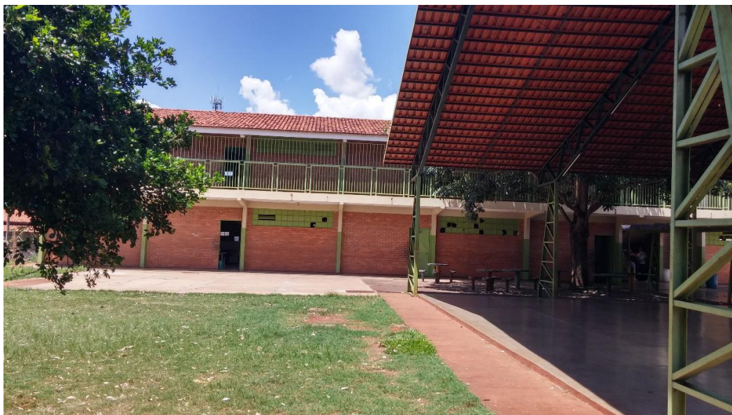
Photograph 1. Block of classrooms where the study was carried out in the public building of teaching.
