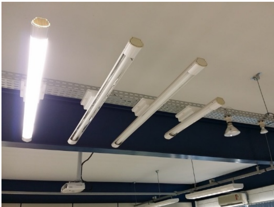
Photograph 4. Set of test lamps installed at LAMQEE.
