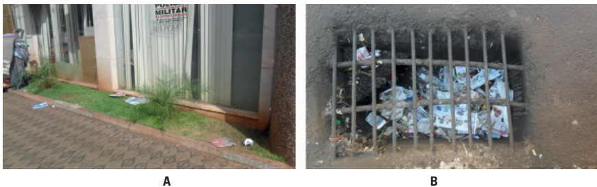
Figure 8 - Effect of inappropriate disposal of SW in the surrounding (A) and in manholes (B)
