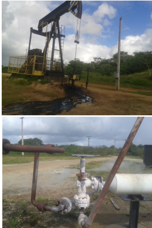
Figure 3 - Oil and gas leakage in the Municipality of Carmópolis, June/2014
